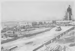
THEN TRUCKLOADS of sand were dumped inside concrete block walls. DESPUES cantidad di truck di santo a worde bashá paden di e murayanan.
